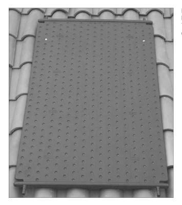
Each collector only needs two rafter anchors on the back (vertical layout).
