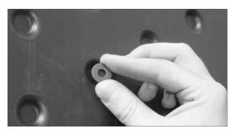
Using the guide plate supplied, drill a hole in the knobs for mounting the collector later.
