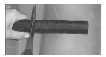
Cut the fabric hoses supplied with the connection and end stopper sets to the length required.
