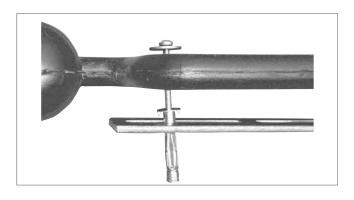
Using a drill with a screwdriver function, tighten the screw, until the plug is properly expanded.
