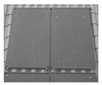
Attach the temperature sensor to the **outside** of the final collector in the collector field (pointing towards the swimming pool). To do this, the temperature sensor can either be attached on site with a Roth pipe attachment adapter or inserted directly into the water using an immersion sleeve.
