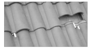
Mount the first rafter anchor on the roof covering. Measure out the position exactly, so that the brackets will be perfectly aligned with the knobs on the collector later. Use this rafter anchor to determine the position of the next one. When determining the position of the second rafter anchor, observe the distance between the knobs, the distance between the potential mounting areas and the width of these areas.
