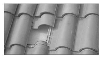
When you have decided where the rafter anchors should be attached, remove the appropriate roof tile. You must choose the appropriate mounting set for your roof tiles.
