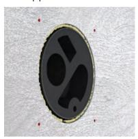
Take the bottom cover of the outside wall panel off again, and prepare a suitable fastening technique for the four fixing points as set out in the façade design.
