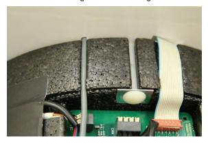
6. After pushing the unit into the wall mounting pipe, connect the plug-in connector part for the connecting cable with the plug-in connector part of the cable for the external control panel.
